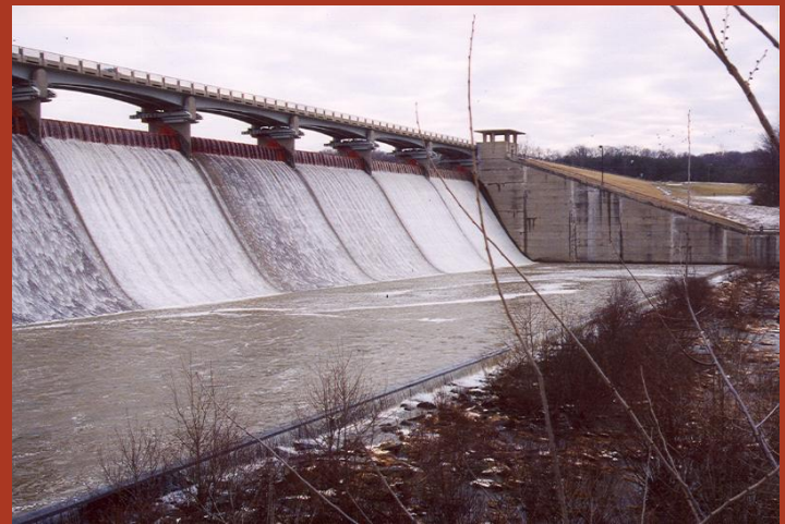
Hoover dam – open locks = released energy
